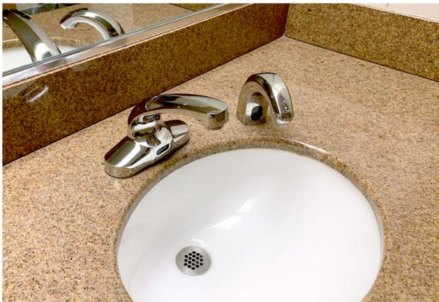
The sensor faucets provide a clean and more modern-feeling restroom experience for building users while helping to conserve water. Since water runs only when needed, sensor faucets can save up to one gallon of water per hand wash.
