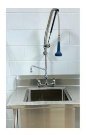
DuraPull features pulldown operation in which users simply pull the sprayer down toward the sink to activate the water flow and release it to end flow. This operational design reduces fatigue and creates a more ergonomic user experience.
